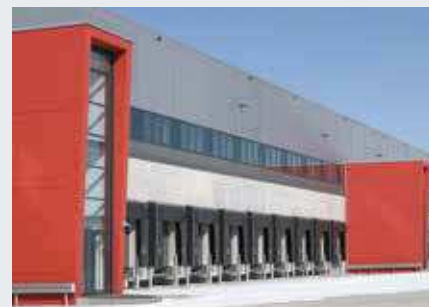
Immogate Logistikcenter, München
